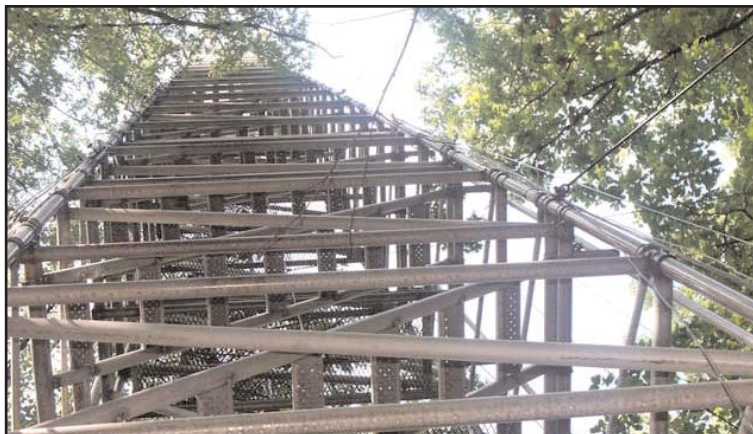
A 100-foot stairway tower similar to this structure at Walker Branch Watershed, Tennessee will provide access to and above the canopy of the forest at BREA. The tower will be instrumented with meteorological and ecophysiological sensors.
